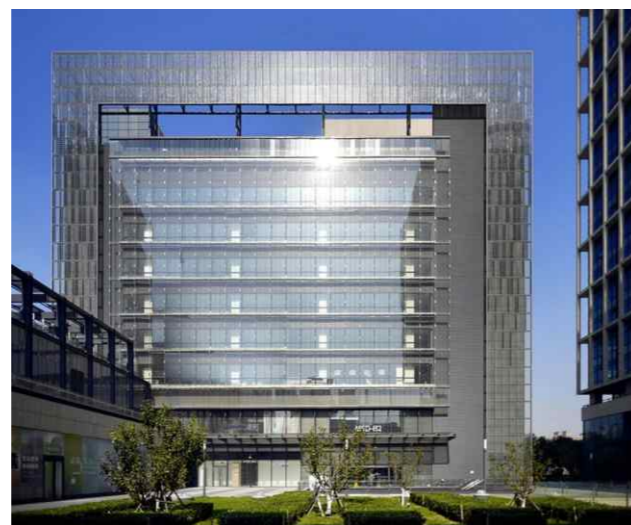
Tianjin Carbon Peaking and Carbon Neutrality Building
